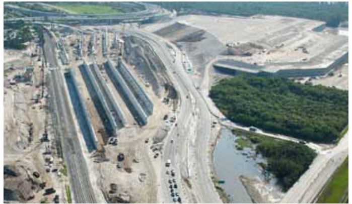
Northeast view of FLL Airport $791 million Expansion showing the U.S. 1 tunnels.
